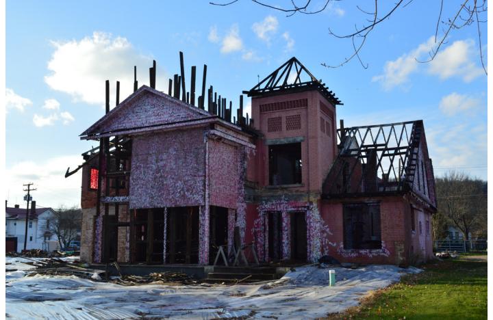
Figure 7: Art installation in progress near Village Hall.
